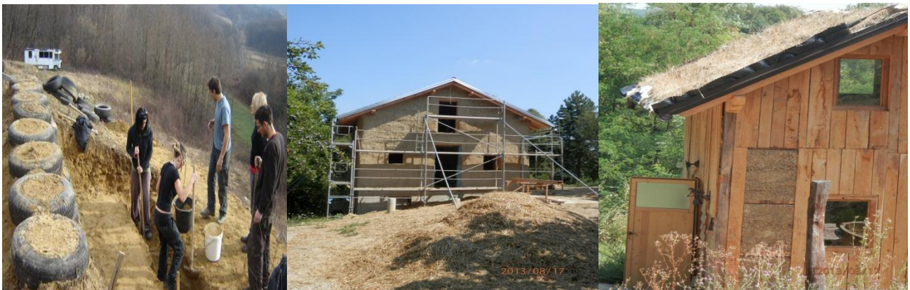
Pictures 4: building the estate of Vukomerić (source: personal photographs; www.zmag.hr )
