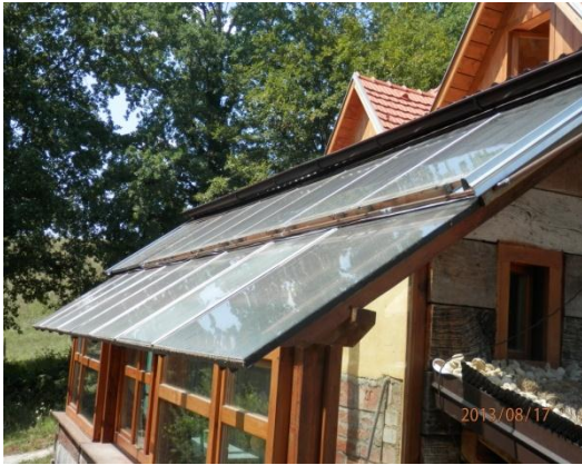
Picture5: solar- panels built by members of association (source: personal photograph)
